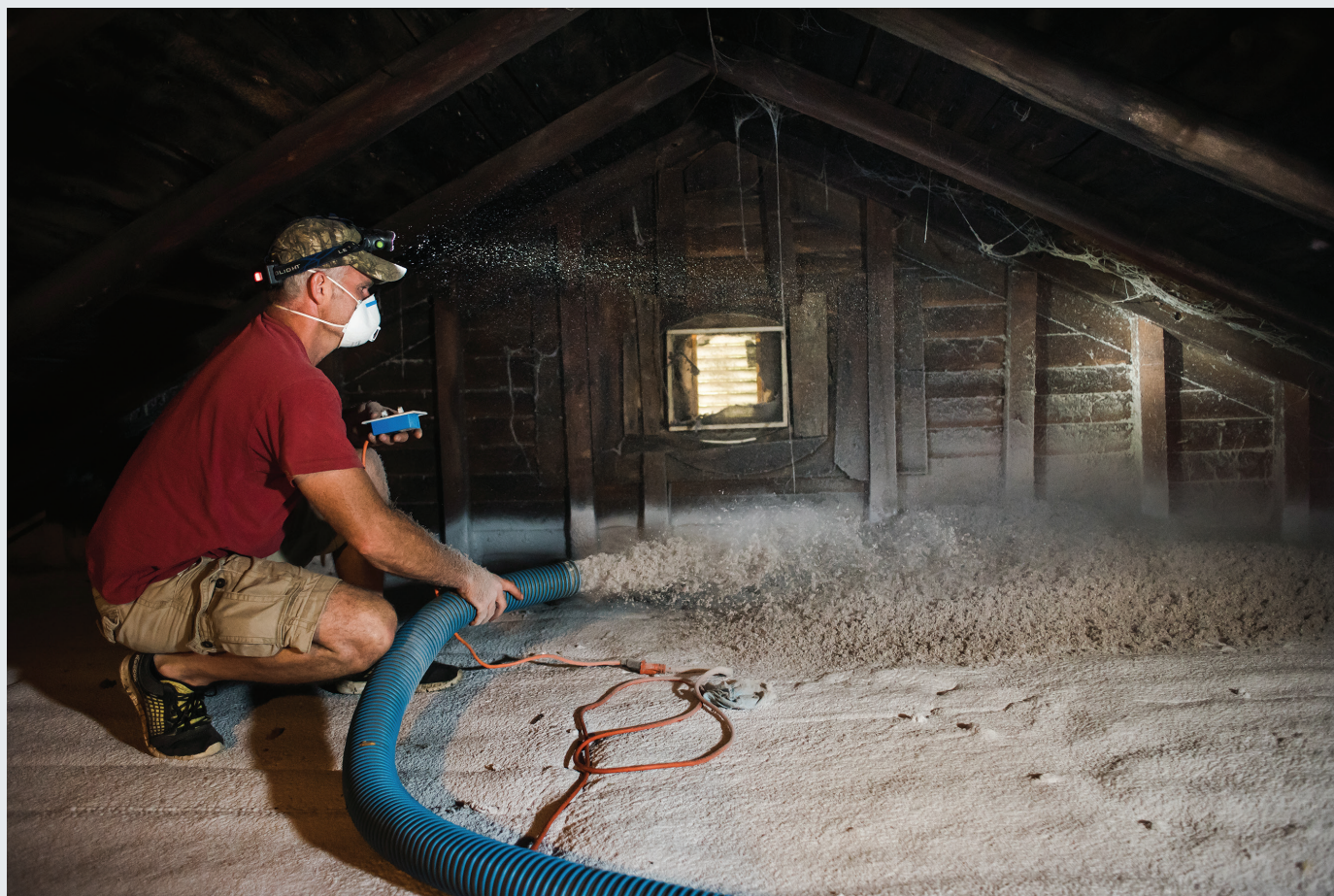
3E Thermal employee adds a layer of cellulose insulation on top of spray foam insulation in the attic of a Middlebury apartment building.
