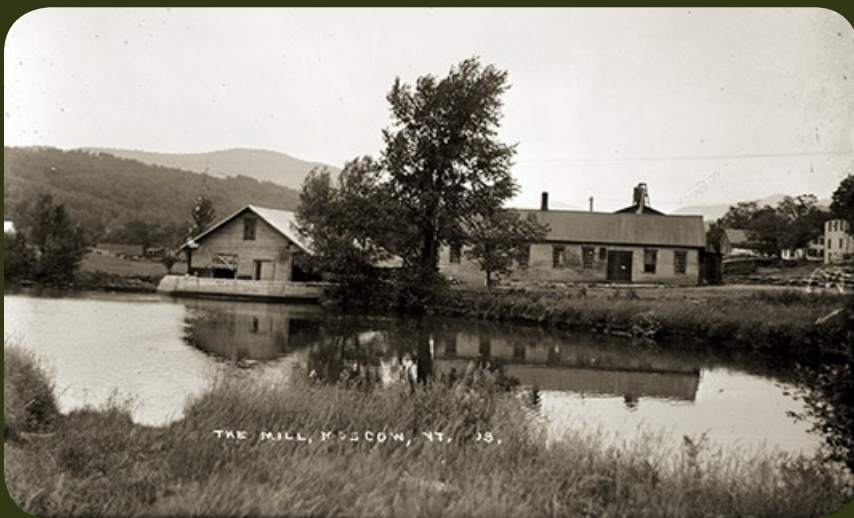
Old Moscow Mill that will be renovated into a modern hydroelectric facility.
